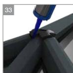
If the project contains central rafters between the hips. Apply a bead of MS polymer around the central bar top cap.
