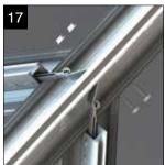
If the project contains jack rafters: Offer up the jack rafter to the hip at the pre drilled holes on the hip rafter, push the bolts through jack rafter bracket and secure with flanged nuts.
