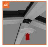
Clip the internal cover up into the ridgeLOCK from below. Ensure clip feature meets the corresponding ridgeLOCK clip feature.
