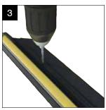
Drill the eaves beam at 100mm from each end and drill a minimum of 4 holes at a Max of 400mm centres using appropriate clearance drill. Now take the eaves beam and ensure correct number of bolts are slotted into eaves beam.
