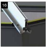
Remove nuts on eaves beam. Fit hip rafters onto bolts at eaves end and hand tighten nuts. Ensure the ridge is now level and using an angle finder check the pitch of the lantern is set at 20°.
