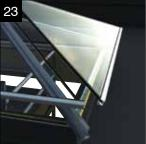
Lower the glass units into place onto the glazing support trim. Ensure that the glass contacts the gaskets on the glazing rafters and the ridge. The glass units should be pushed up towards to the ridge as far as they will go.
