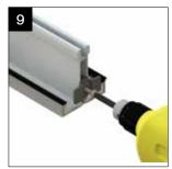
Attach the glazing rafter end cap brackets - as access restriction may prevent easy fixing later.
